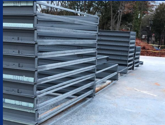
All hollow-metal frames for lower level masonry walls on site
