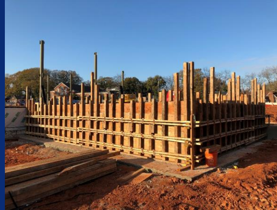
Forming in place for south stair tower foundation wall
